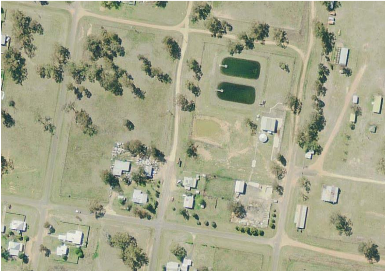
Figure 36: Mendooran WTP site
