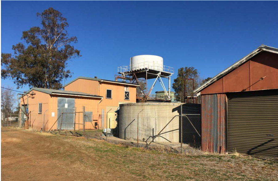
Figure 2: Baradine WTP, Walker Street and Baradine Road
