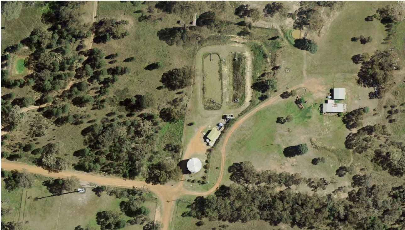
Figure 18: Binnaway WTP site
