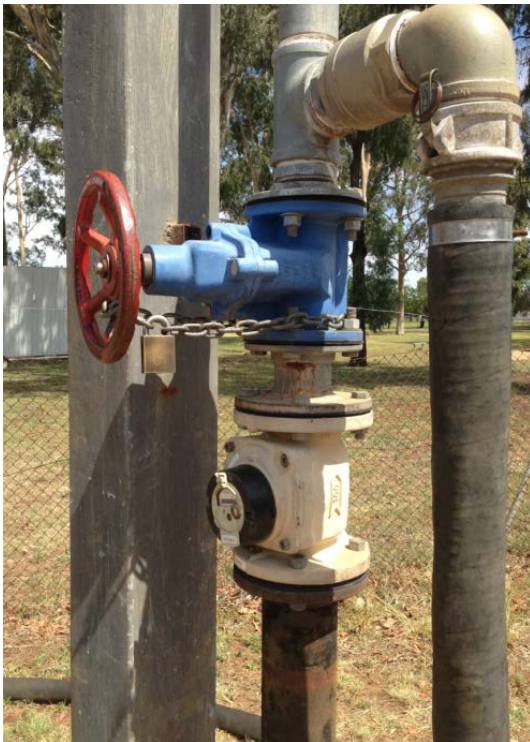
Figure 10: Gilgandra standpipe
